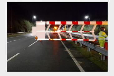
Kier is trialing a new gate system on a road job in Surrey which is designed to replace rows of cones to taper off lanes and protect highways workers. The SwiftGate system can be fully deployed in five minutes compared to the 25 minutes it takes road workers to put out the taper of cones directing often fast-moving traffic away from a live lane.
